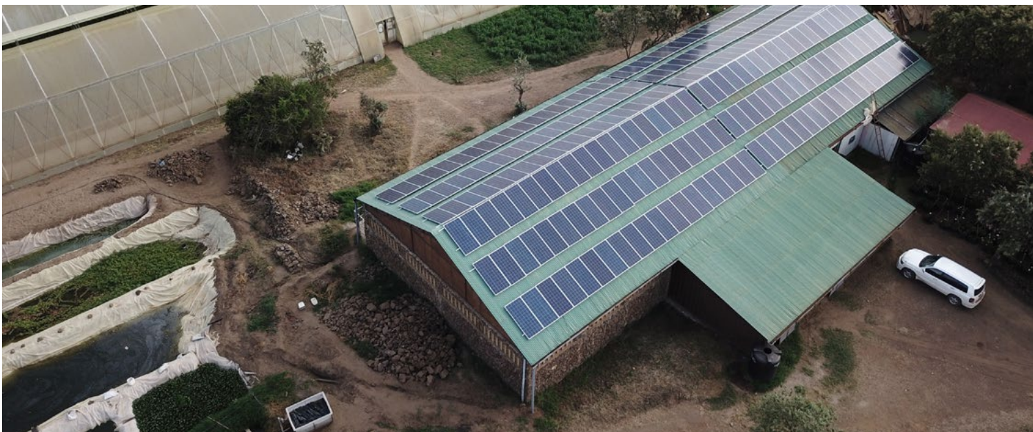
Roof mounted solar power plant on a rose farm in Kenya.
